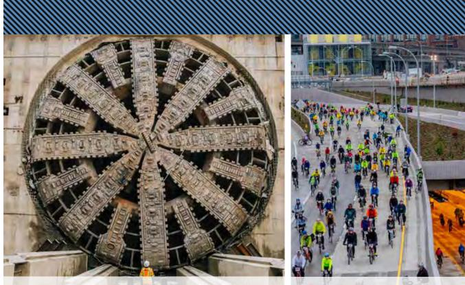
The tunnel boring machine, "Bertha," breaks through into the receiving pit at the end of the SR 99 tunnel.
